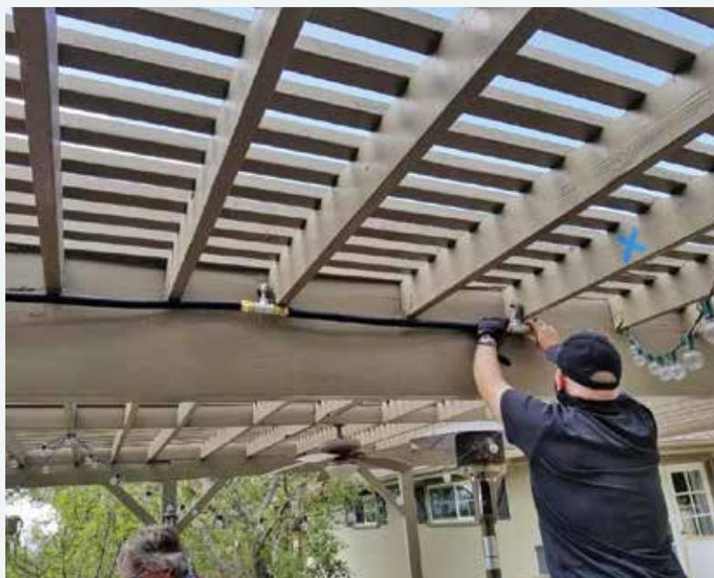
Corrugated Stainless Steel Tubing, or CSST, is an ideal match for outdoor rooms because its flexibility allows it to be installed in a variety of configurations to meet design needs.
